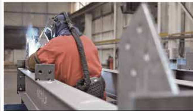
OLD WAY - Manual Tacking and Welding
